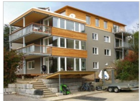
Multi-family house in Zurich-Hoengg. The building was not only insulated with prefabricated elements, the old balconies have been replaced by larger ones in front of the building and are now used as living room extensions. In addition, the unused roof space has been replaced by an attractive apartment (Architect: Beat Kaempfen, Zurich).
