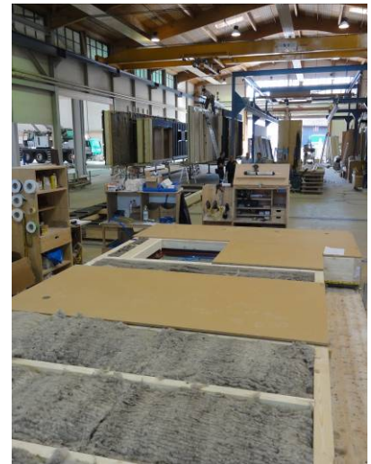
Figure 13: The insulated timber frame construction is closed with a medium dense fibre board.
