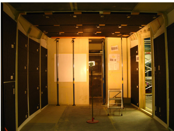
Figure 5: Insulation works with Aerogel blankets and vacuum insulation panels (VIP) at the inside of space unit 1
