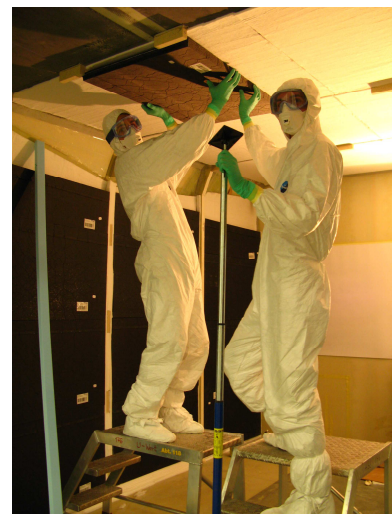
Figure 5: Insulation works with Aerogel blankets and vacuum insulation panels (VIP) at the inside of space unit 1
